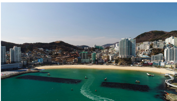
Photo 1. Submerged breakwaters to protect beach erosion of Songdo, Busan ( https://www.crowdpic.net ).
